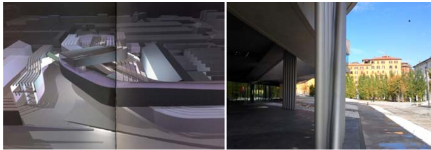
Figure 6 Design when Procedure Realm prevails - New seismic codes forced to cut squared shaped wings in smaller parts so that unforeseen pillars had to be built to sustain them. MAXXI museum, Rome, 1999 - Z. Hadid
